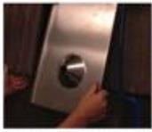
With wedge still in place on the leading edge of tiles above, lift left side tile and set aluminum flashing into place.
