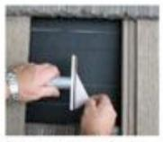
Remove protective paper from bottom of post base and place onto centermarks.
