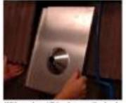
With wedge still in place on the leading edge of tiles above, lift left side tile. and set aluminum flashing into place.
