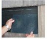
Remove post from plate, instal "peel and stick flashing" over plate with stud protruding through hole
