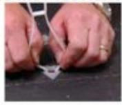
Remove Plate, drill 3/4" hole through deck. Insert toggler bolts per Toggles Instructions.
