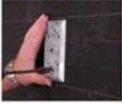
Use the Mounting Base as a template Measure up 6 5/8" to center of mount. to mark the drilling of the top and bot-
