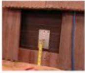
Remove Tile at location of Mount. Mark paper, then measure 5 1/2" from tom holes. exposed edge of adjoining right tile to center of mount, and mark paper.
