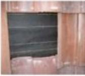
Remove Tile at Location of Mount Installation. Locate center of rafter and mark with a sharpe pen
