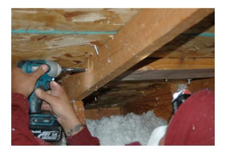
Lag bolts into the deck must go into **plywood** thicker than 1/2" 1/2 OSB calls for toggler bolts or putting in blocks for lags
