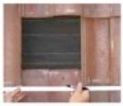
Use a straight edge and measure up 6 5/8" from bottom of tiles to center of the post, over the center of rafter.
