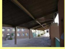
This almost football field long project is a dual purpose design serving as a shade structure over a 20' wide walkway extending between pool community center and clubhouse. The corrugated metal roof with its south by southeast orientation is pitched at 17 degrees and supports 106 unglazed 4' x 8' pool solar collectors totaling 3,392 sq. ft. The balance of the structure is fabricated in metal with the exception of pre-existing decorative pillars supporting the trailing edge of the roof structure.
