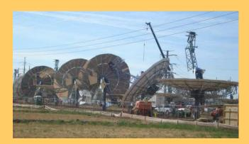
A: They are Tessera Solar's 1.5 MW Dish Stirling solar farm. The mirrors concentrate the sun's energy onto a Stirling heat engine which in turn powers an electric generator. There will be 60 dish/engine units at the site when it is completed early next year.
