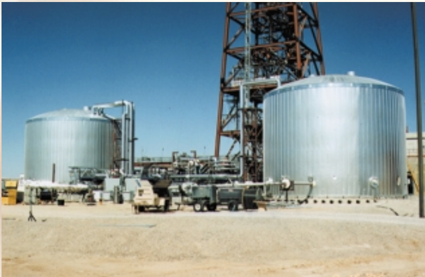
The thermal storage system at Solar Two. Pictured are the 230,000-gallon hot (left) and cold (right) salt storage tanks. The steam generator is in the center. These high-temperature tanks are the largest of their kind in the world.
